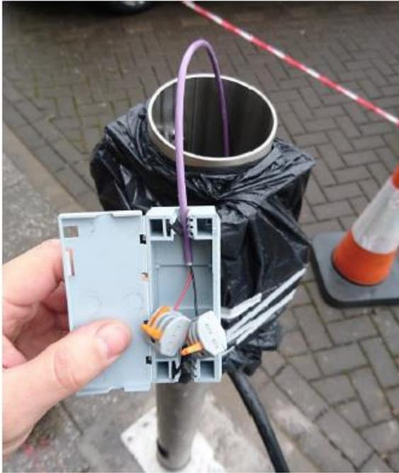
Figure 2 - Wago connectors linking up the serial bus
