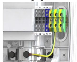
Figure 8: Securing the ground
